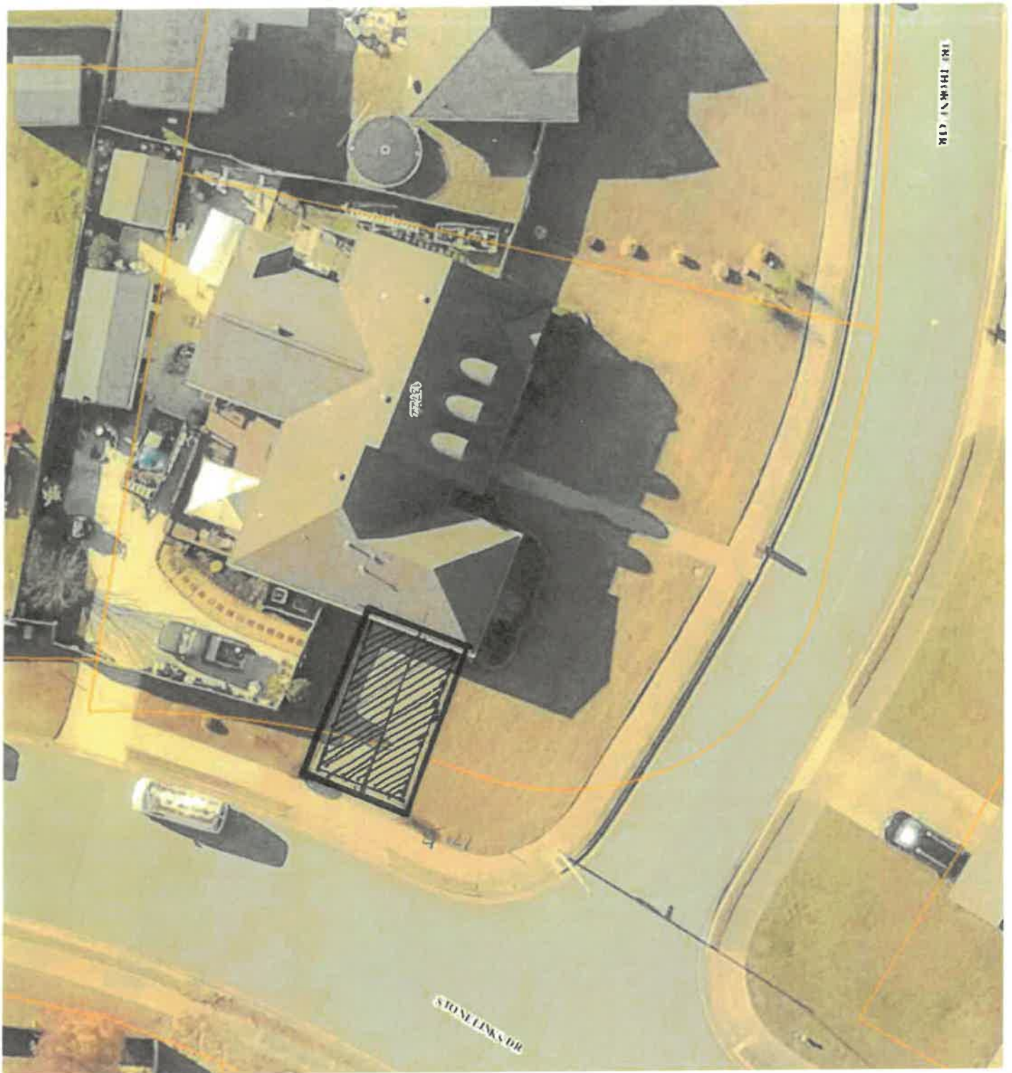
Approximate Size and of Location Carport as Constructed
