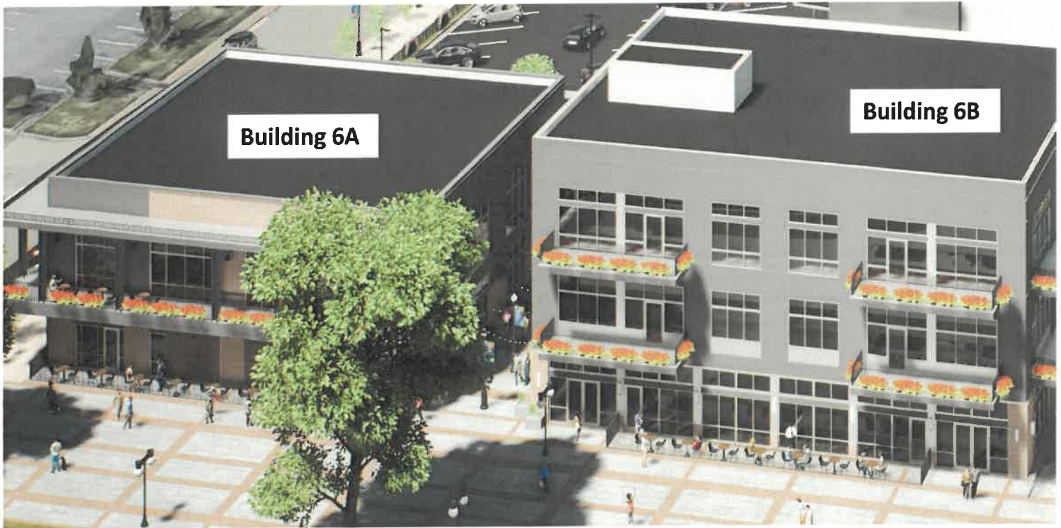
Zoomed View of south sides of Buildings 6A & 6B showing patio space
