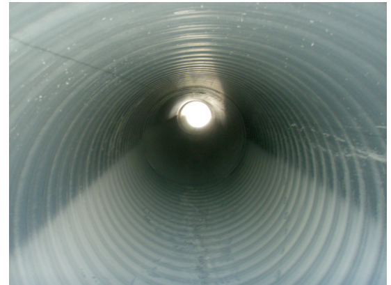
Smooth Interior Wall
