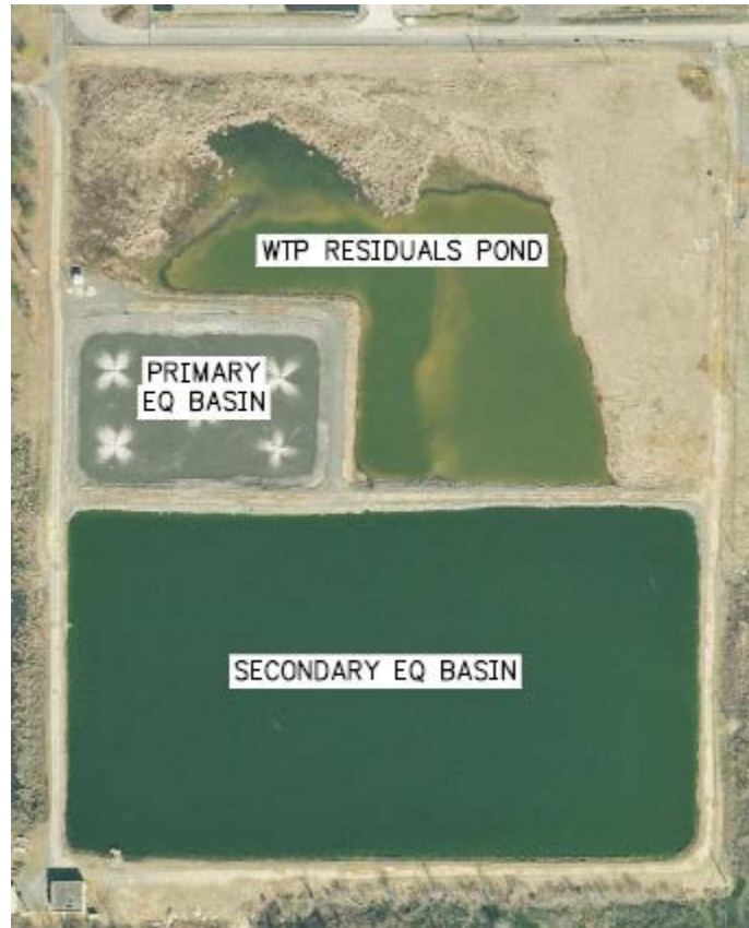
Exhibit 3.3 – Aerial Photo of WWTP Ponds
