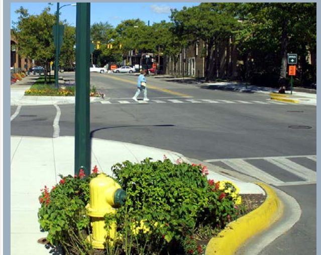
A curb extension in Birmingham, AL shortens the crossing distance for pedestrians
