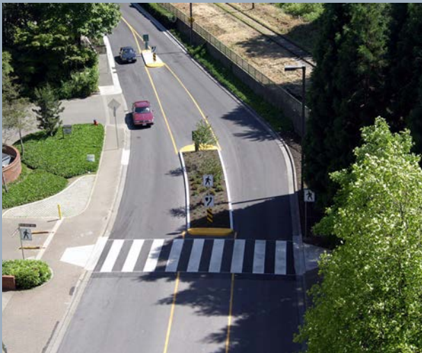
Crossings must be located where there is a strong desire to cross and where sight distances are good
