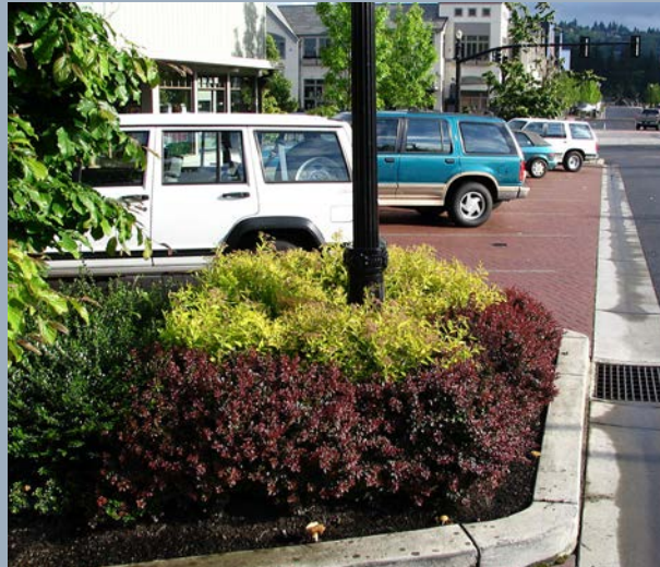
Sudden downpour can create flash flood conditions. Valley gutters and rain gardens help channel water away from pedestrians
