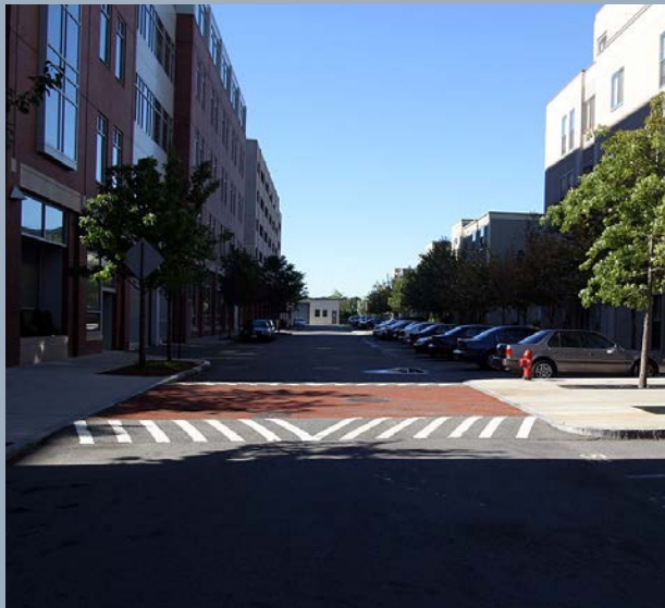
A raised mid-block crossing in Cambridge, MA helps motorists see pedestrians in deep shadow
