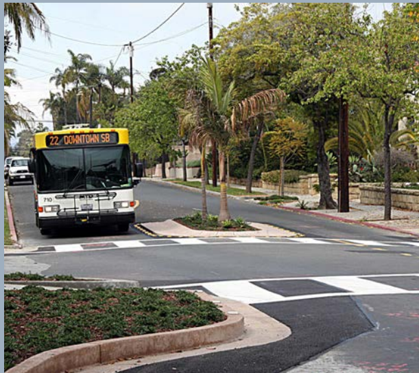
A large vehicle being deflected through a neighborhood Intersection Chicane, Santa Barbara, CA
