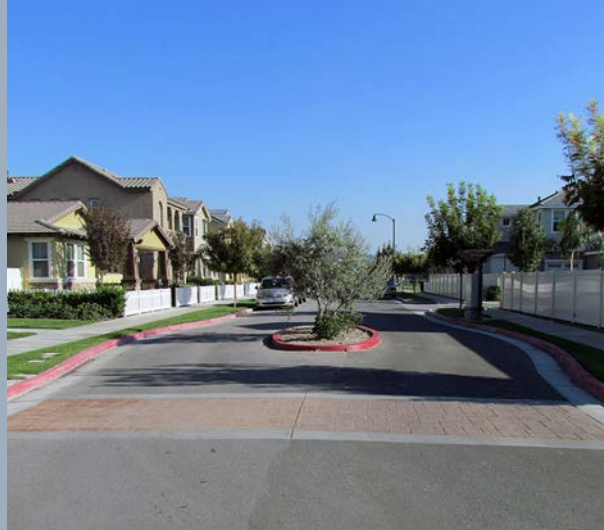
A short median in Loma Linda, CA announces the entrance to a residential neighborhood
