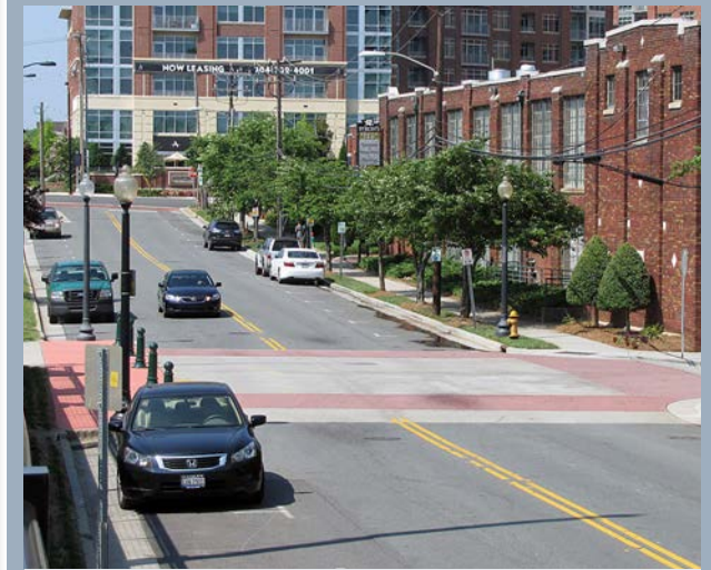
Raised intersections bring speeds under control and help motorists and pedestrians see each other
