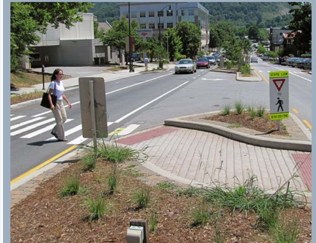
Pedestrian refuge islands buffer pedestrians from traffic, allow crossings in stages and angle pedestrians correctly to face traffic.
